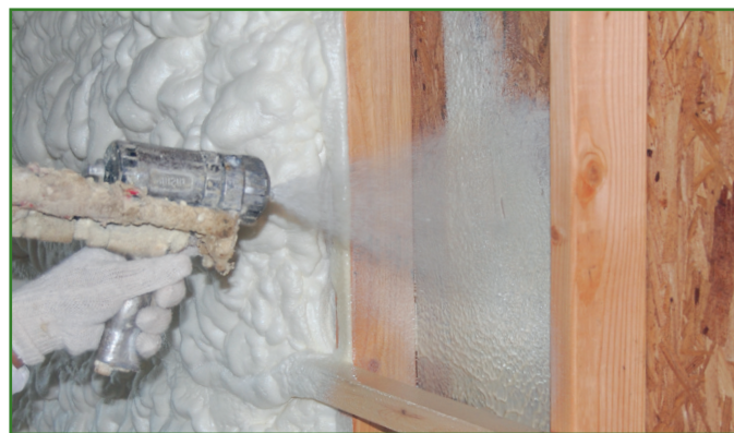
BioBased Insulation® being applied
